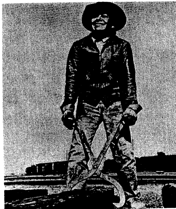
Figure 3-16. Handling treated wood ties.
