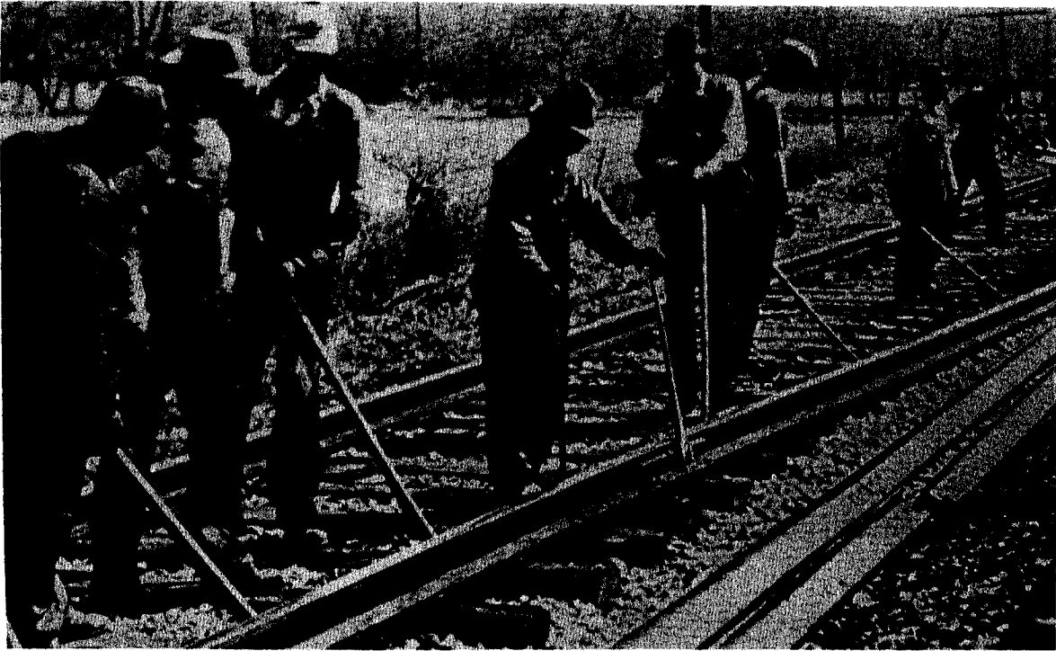
Figure 3-36. Rail being lined out.
