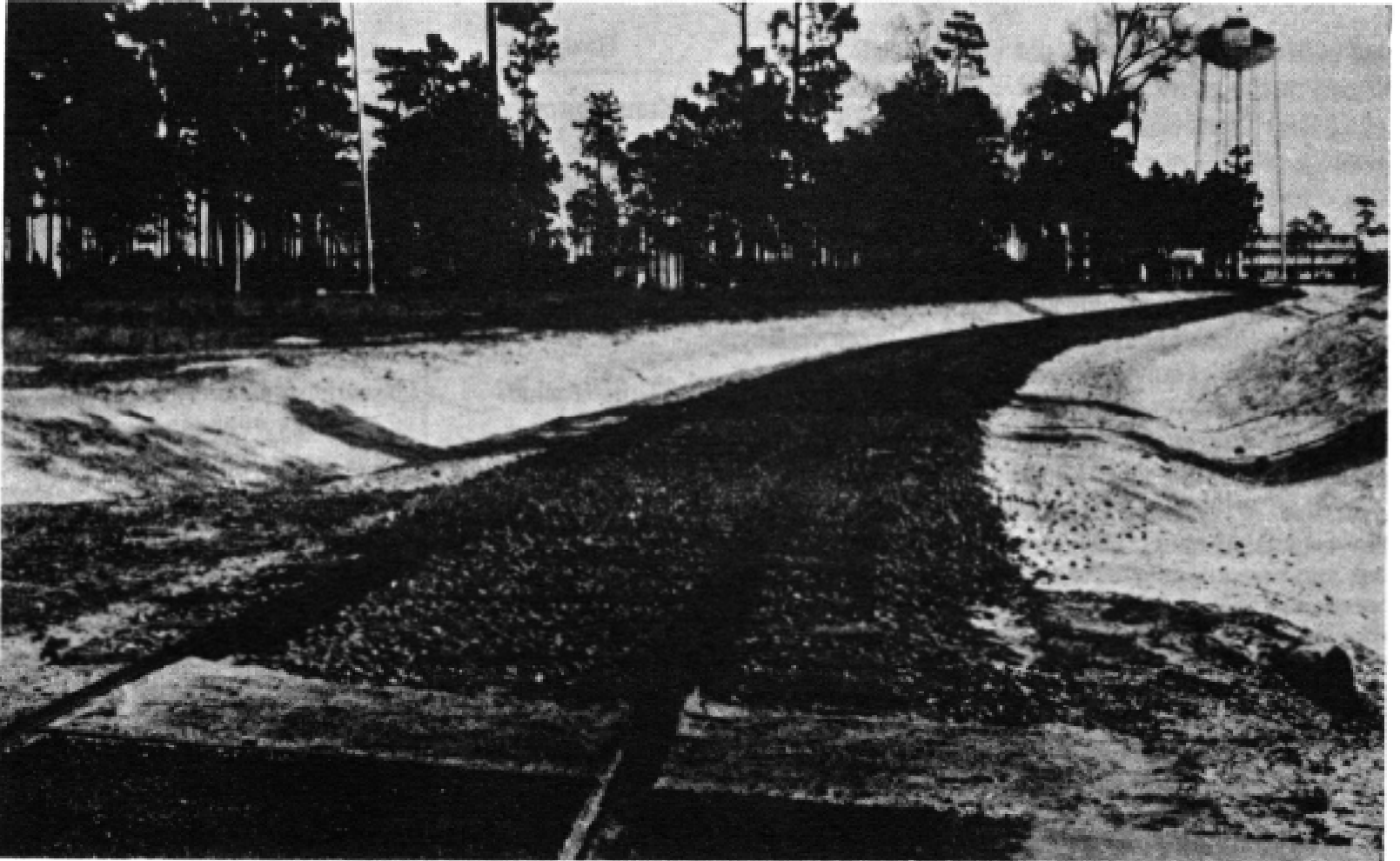
Figure 1-1. Example of well-maintained track.
