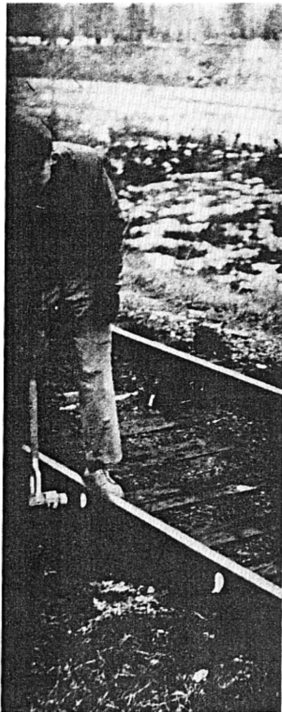
Figure 3-21. Spot marking rail with paint.
