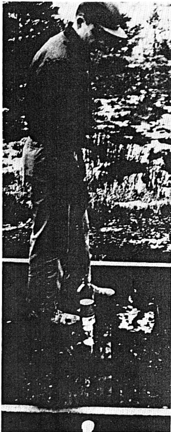
Figure 3-20. Spot marking ties for removal.
