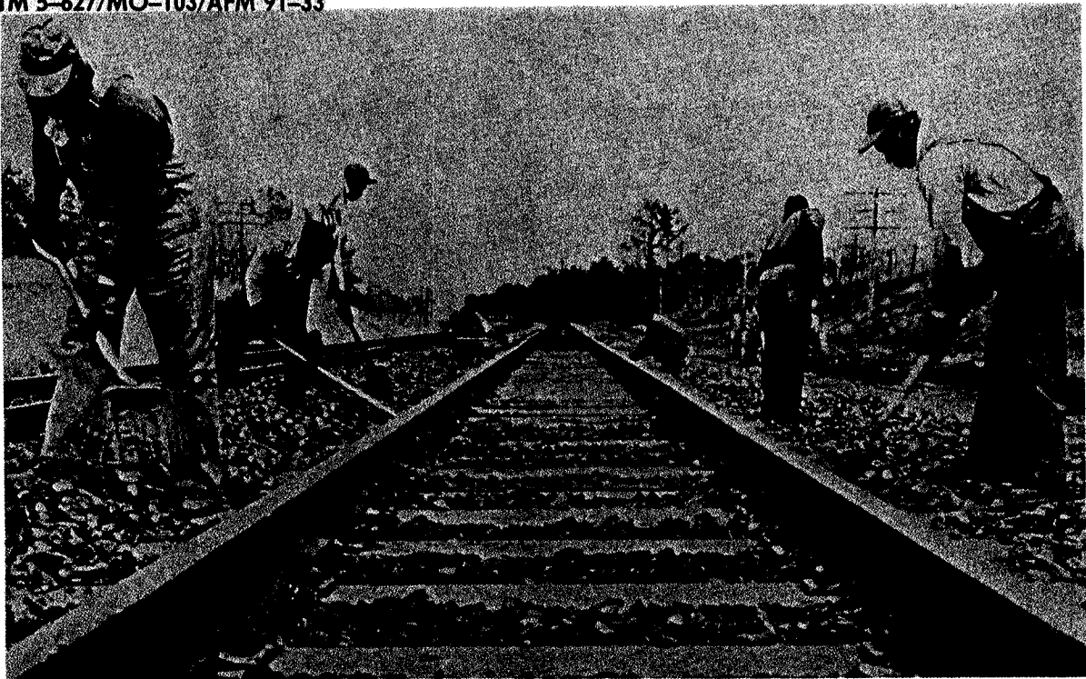
Figure 3-6. Hand-placing ballast after mechanical distribution.
