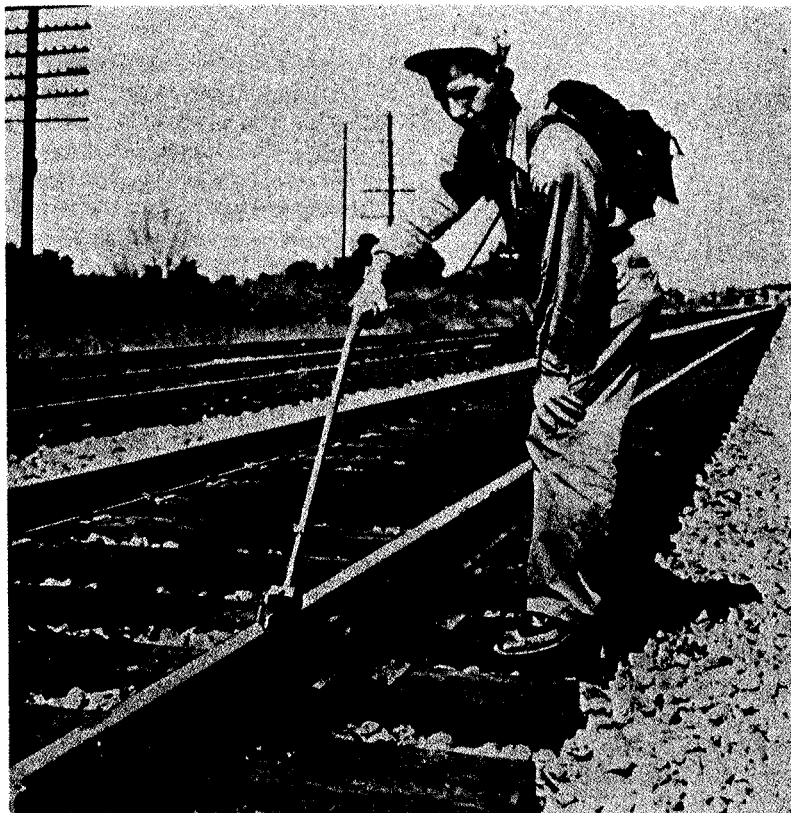
Figure 3-25. Inspecting rail for flaws with a sonic detector.
